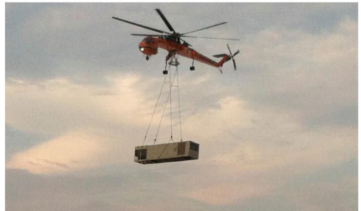
The helicopter positions a 90-ton Daikin RoofPak unit for the expansion facility—17 units set within 90 minutes
