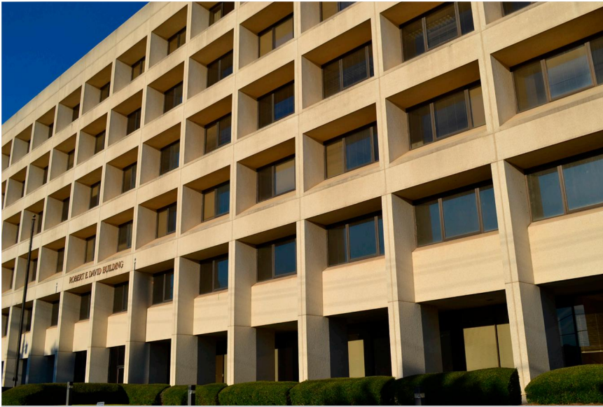
The Robert E. David building is home to South Carolina's Department of Employment and Workforce agency which recently upgraded its original 1975 chiller system to increase energy savings.
