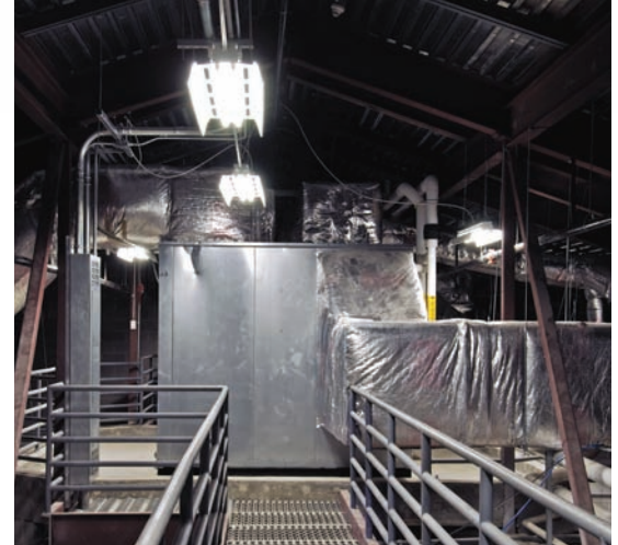
Greenheck's Energy Recovery Units, Model ERCH, installed at Rockingham School.
