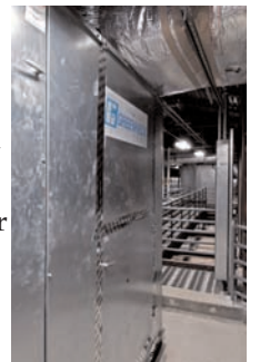
Greenheck's Energy Recovery Units, Model ERCH, installed at Rockingham School.
