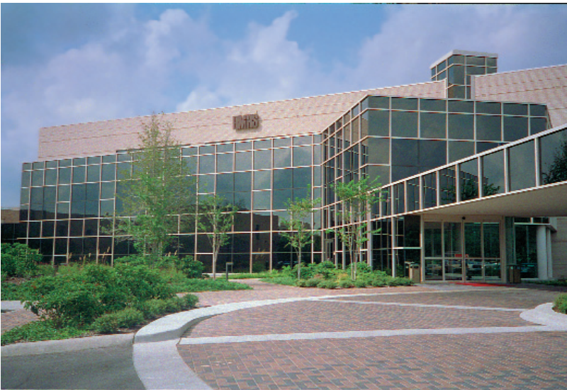
At Northeast Baptist Hospital, a MDAire desiccant system allowed major improvements in comfort control for the operating rooms. The entire project was completed without a single interruption of surgery schedules.
