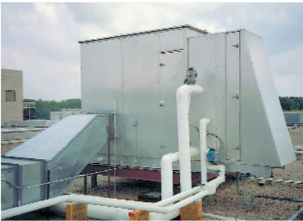
*Because the MDAire system was installed on the roof and connected at the fresh air inlet, it was easy to retrofit and upgrade the old HVAC system without interrupting normal hospital operations*
